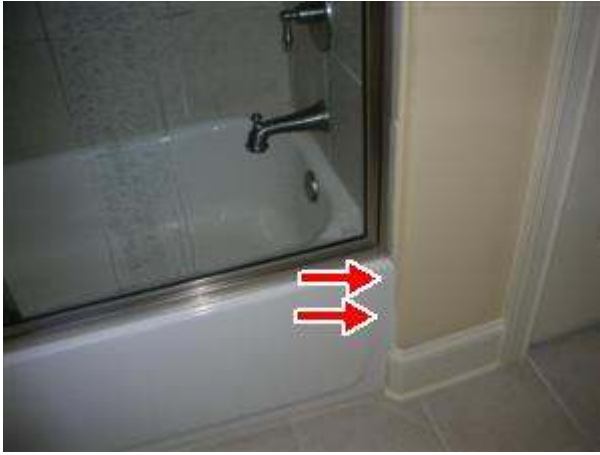
E. Picture 2 third floor bathroom
