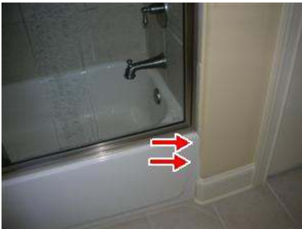
E. Picture 2 third floor bathroom
